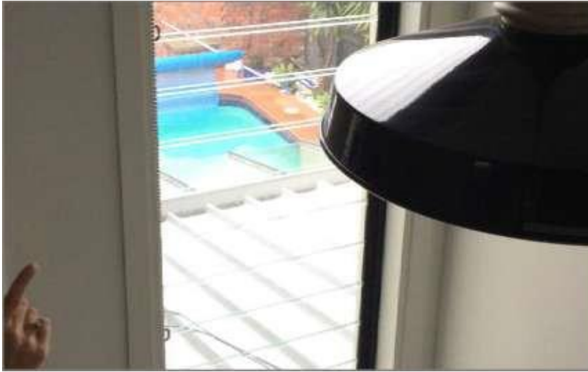
Image: New window in good condition.
