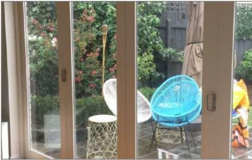
Image: New bi-fold doors in family room in good condition.
