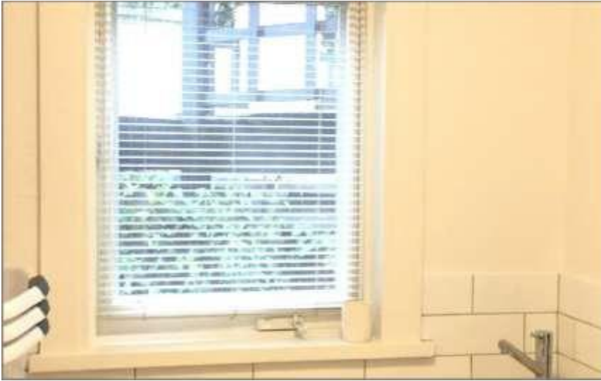
Image: New windowing laundry in good condition
